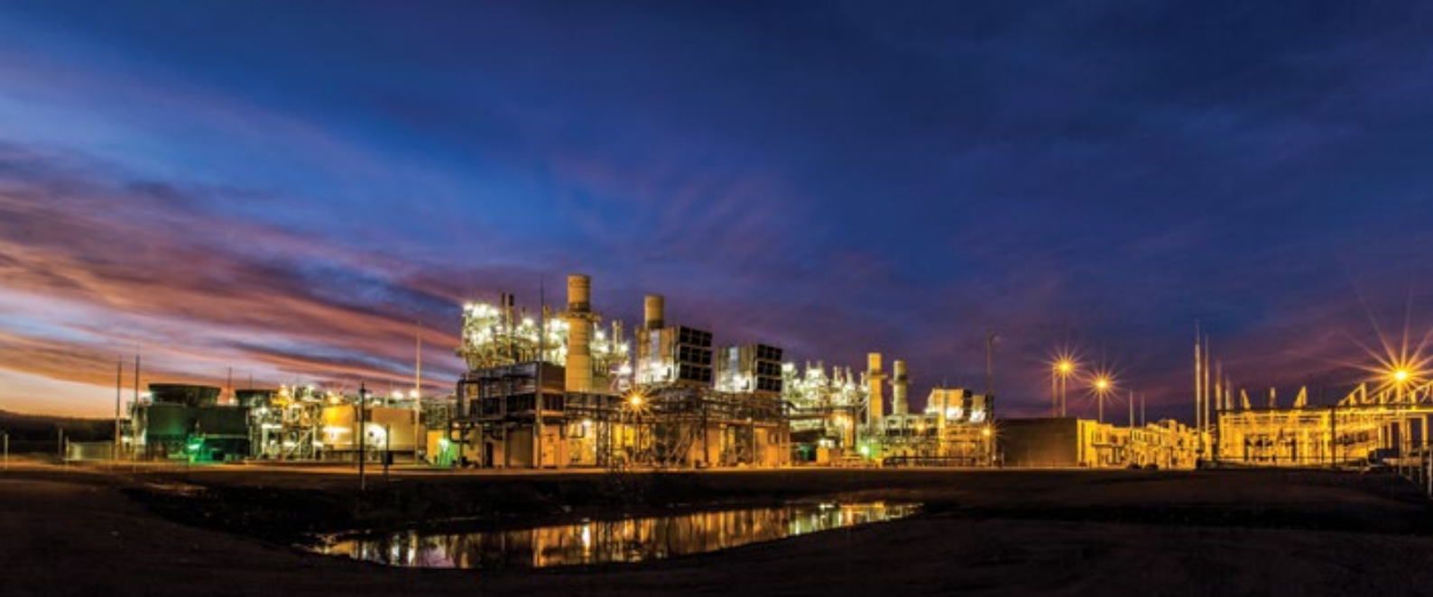
Diamantina Power Station commenced supplying gas-fired power to North west Queensland in FY2015
