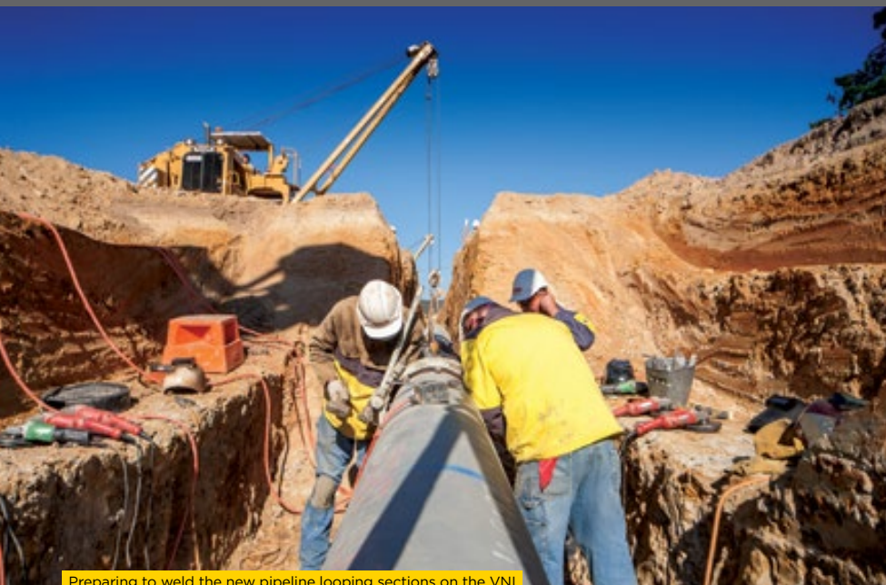
Preparing to weld the new pipeline looping sections on the VNI
