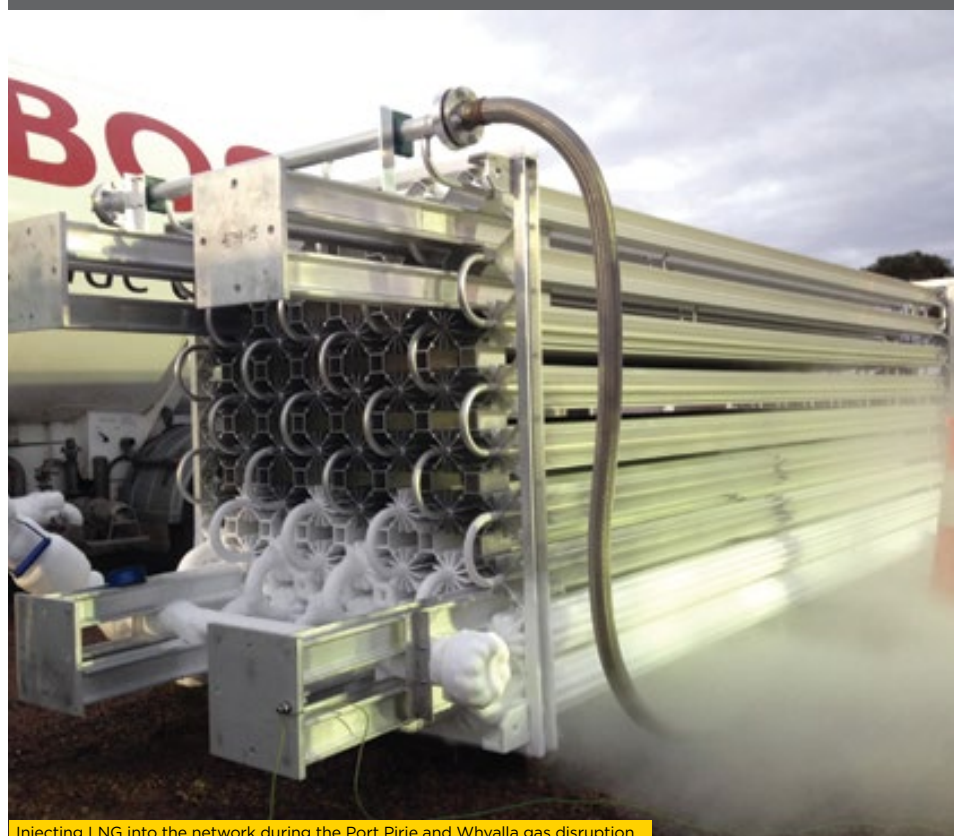
Injecting LNG into the network during the Port Pirie and Whyalla gas disruption
